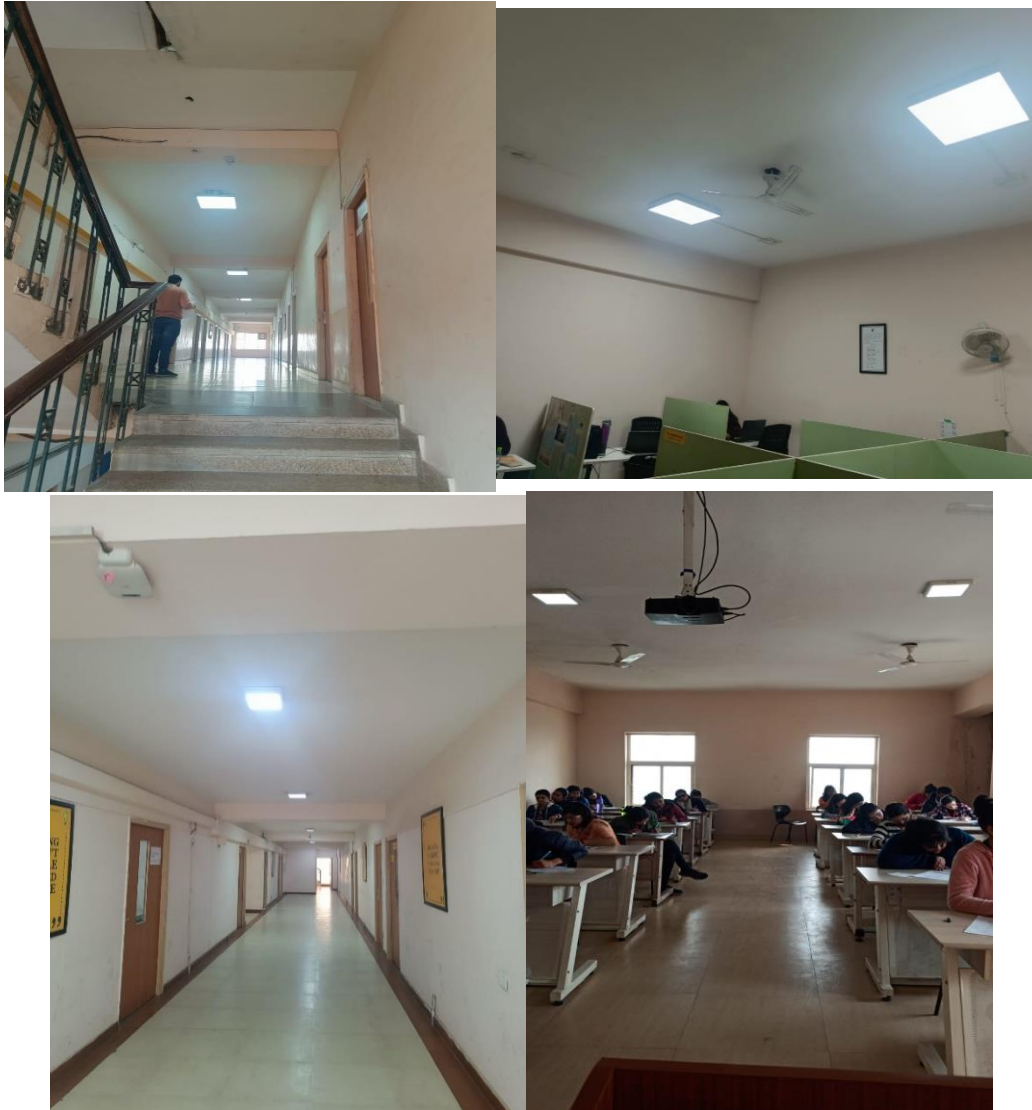
Installation of LED Lights
